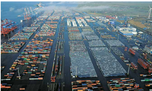
Container Terminal CT IV
