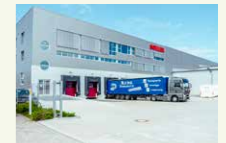
SOLLER, Bremen Industrial Park
