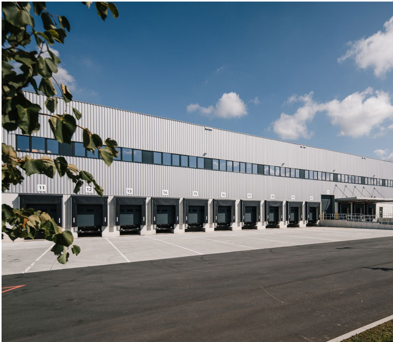
L.I.T. AG, CARGO DISTRIBUTION CENTRE BREMEN (GVZ)
