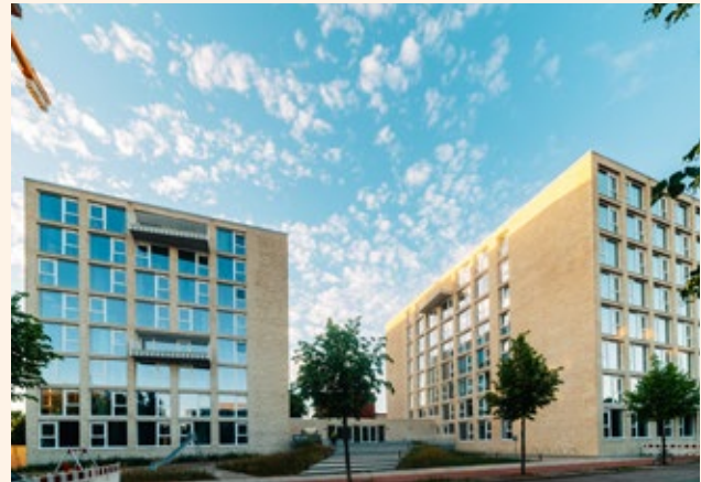
Student residence, Technology Park
