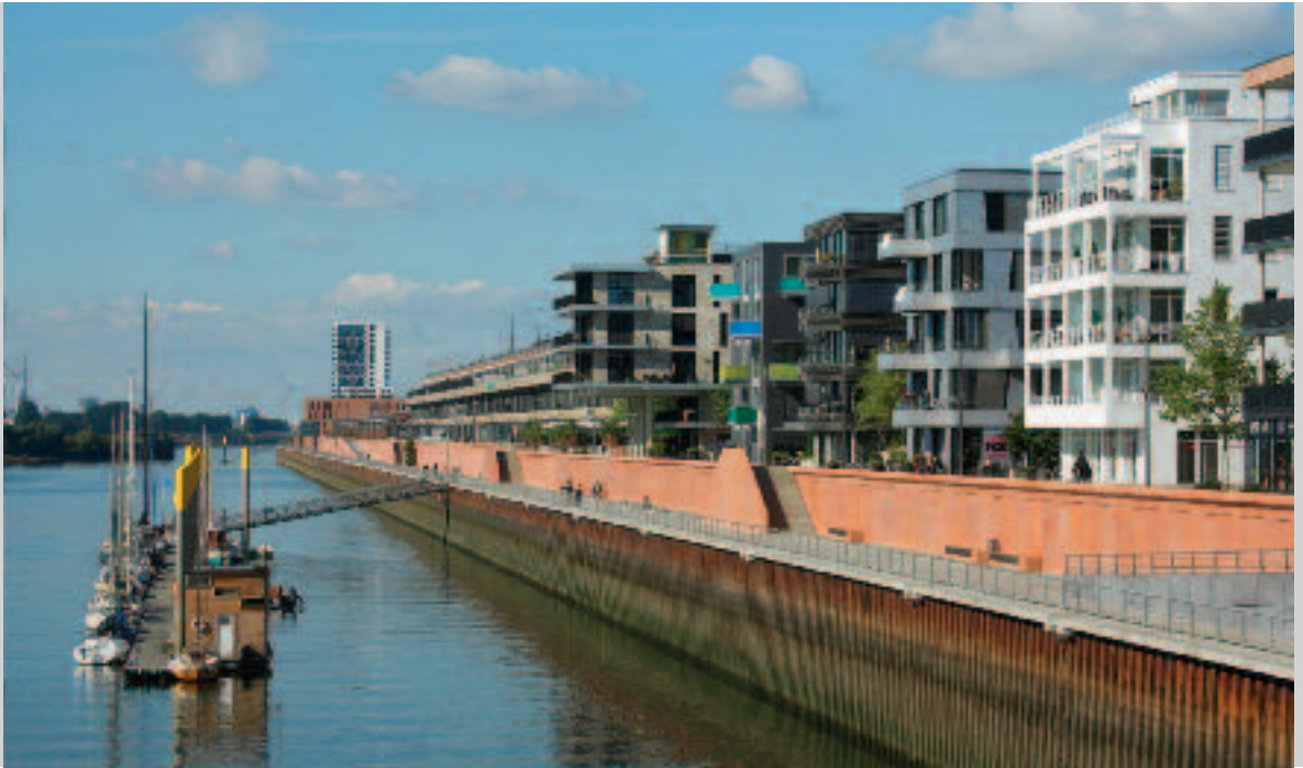
Europahafen: where high-tech engineers work next door to whisky distillers, yacht chandlers, fashion designers, silversmiths and film producers. The city's biggest restaurants can also be found here.
