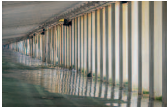
The columns take the force out of any storm surge.
